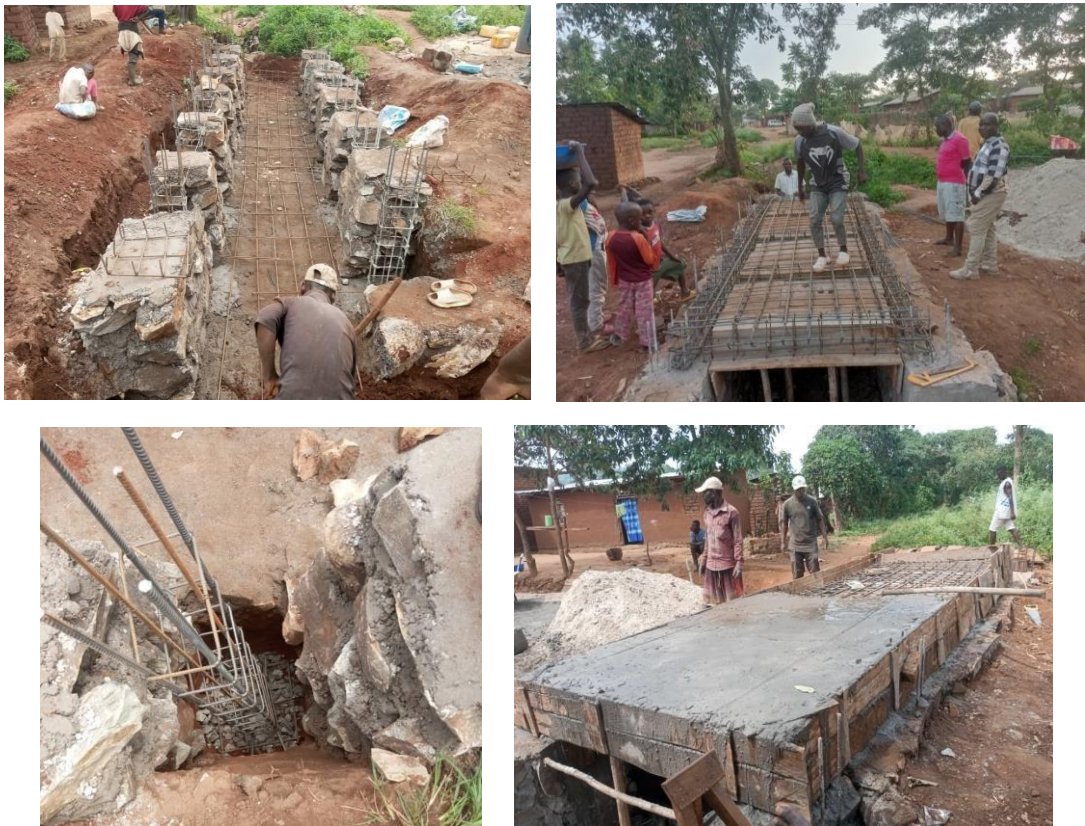
Photos : the different stages of the bridge construction
